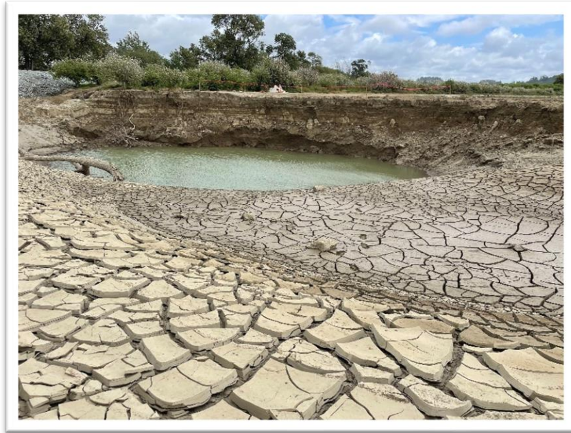
Figure 7. Erosion on Willoughby Farms' O'Connell Ranch caused by Levee breach.
