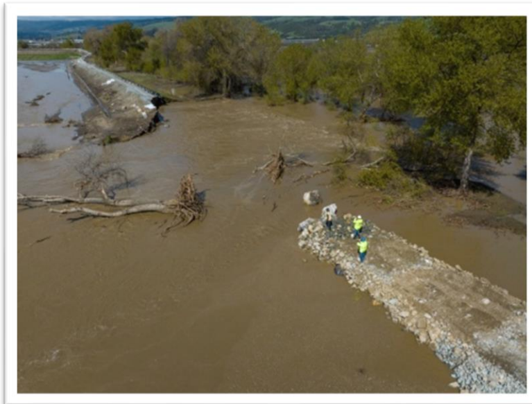
Figure 5. The Pajaro River Levee Breach. Source Ken James, Department of Water Resources, March 13, 2023, published at Monterey Herald .
