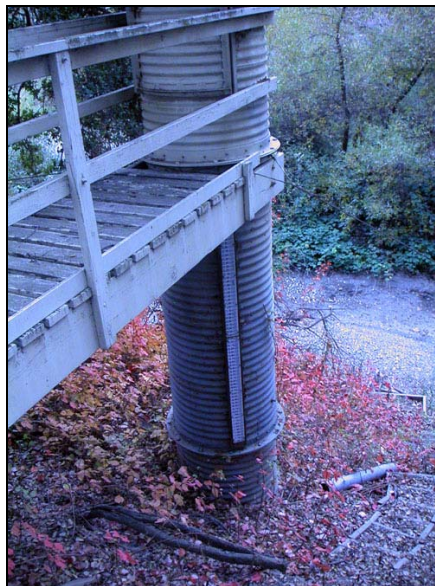
Figure 10: View of Pacheco Creek stilling well structure.
