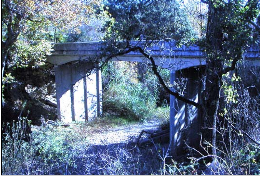
Figure 8: Walnut Avenue Bridge (facing downstream)
